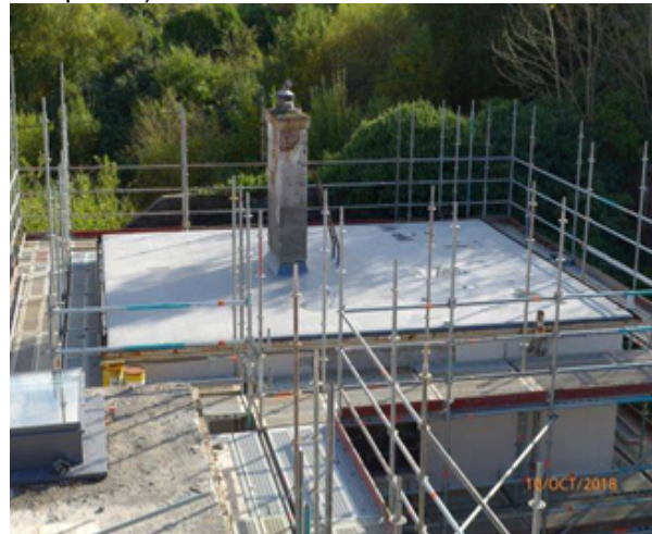
Looking South: General View of Caretakers House Roof (NB: gutters yet to be replaced).
