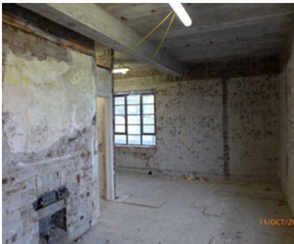
First Floor: General View.
