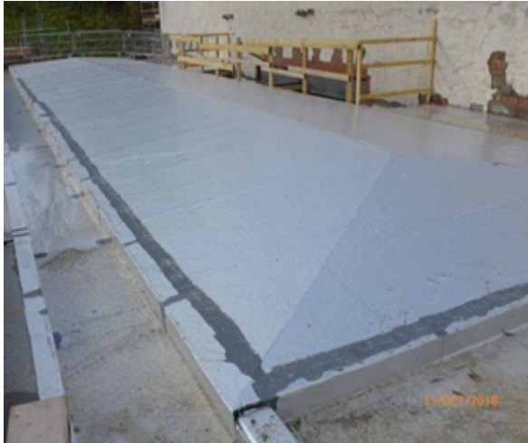
Looking West: new Roof over First Floor Offices & RPM Studio.
