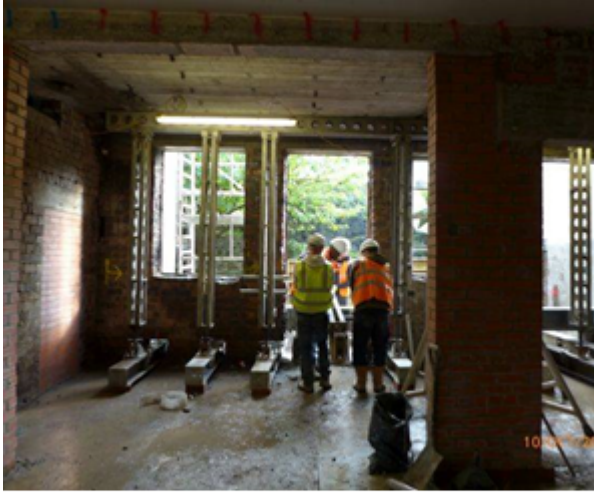
Shop Area (NB: Work in Progress: temporary property in preparation for demolition of existing external wall – new structural steel beam visible at ground level).
