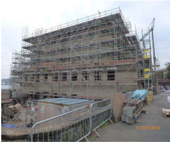
North Elevation (Mackinlay St.).
