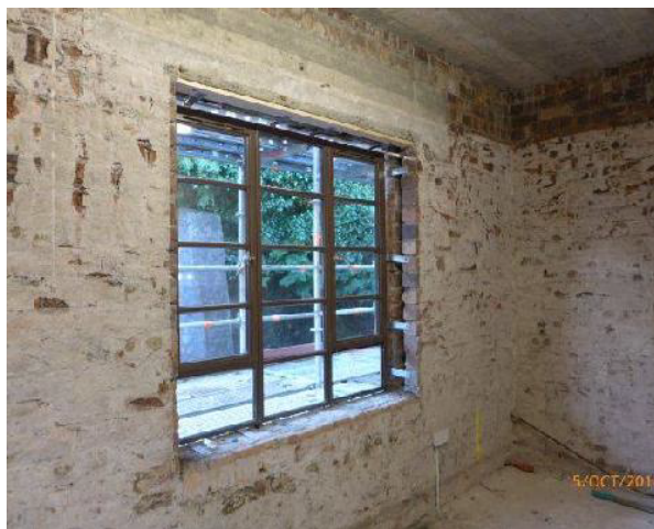
South Elevation: new window to first floor office area now installed.
