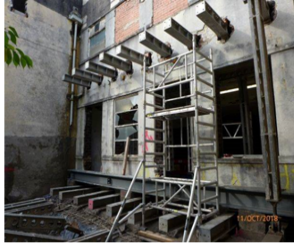
Shop Area (NB: Work in Progress: temporary property in preparation for demolition of existing external wall – new structural steel beam visible at ground level).
